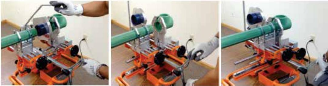
Picture no. 39: Welding and cooling of pipes and fittings
