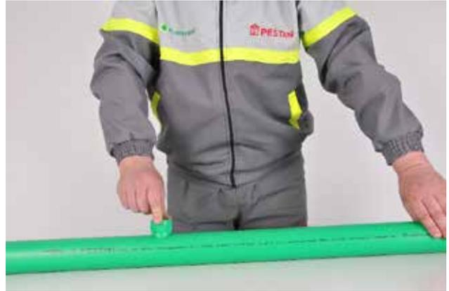
**Picture no. 29:** Insert the saddle coupling on the wall of the pipe
