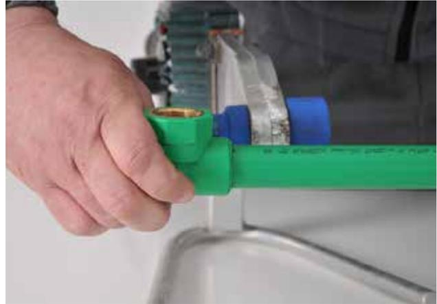
Picture no. 25: Connecting pipes and fittings
