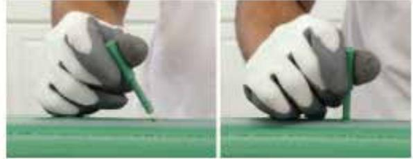
Picture no. 48: Inserting the repacking plug
