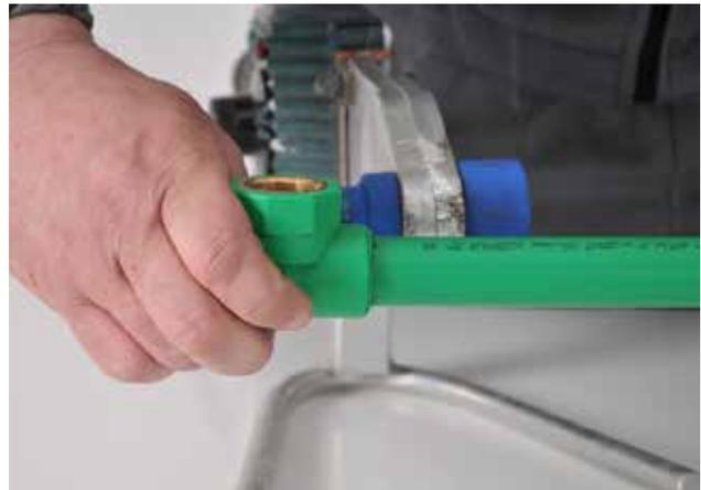
Picture no. 25: Connecting pipes and fittings
