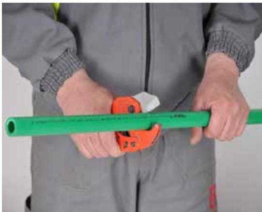
Picture no. 19: Cutting PP-R and PP-RCT pipes
