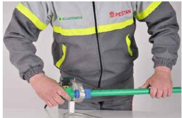
Picture no. 23: Heat pipe and fittings (pay attention to positioning the pipes and fittings on the heating plate)
