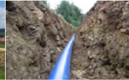
Installation without sand bedding
