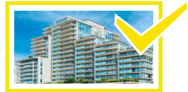
Hotels, hospitals, residential complexes
