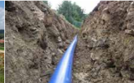
Installation without sand bedding
