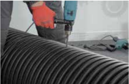
3. Drilling holes for the guided crown saw
