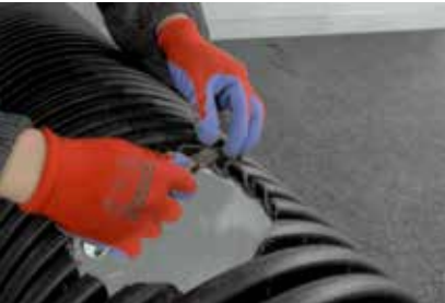
5. Cleaning chips and forming a clear hole
