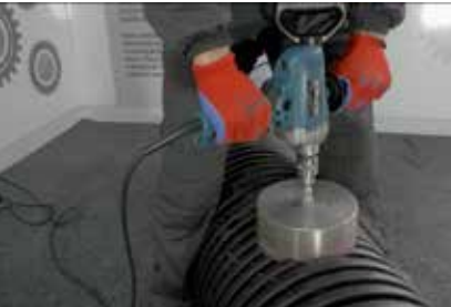
4. Drilling holes with crown saw
