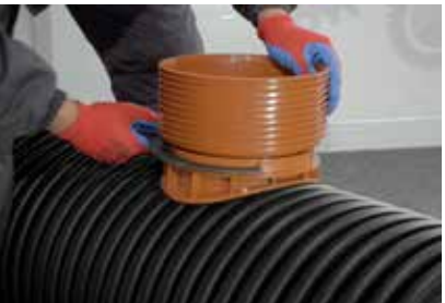
12. Final tightening of sag
