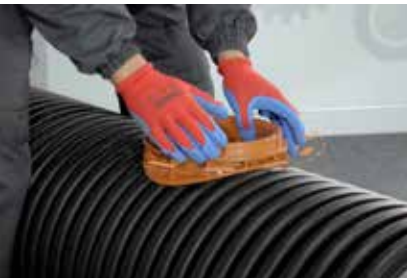
9. Tightening the sag
