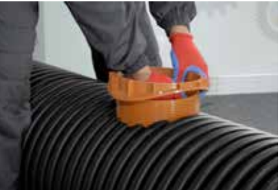
8. setting the spacer ring
