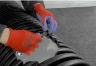
5. Cleaning chips and forming a clear hole
