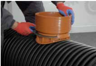
12. Final tightening of sag
