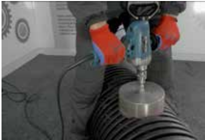
4. Drilling holes with crown saw
