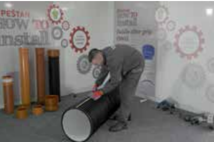
2. Determining position for montage
