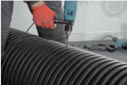
3. Drilling holes for the guided crown saw
