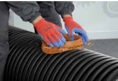
9. Tightening the sag
