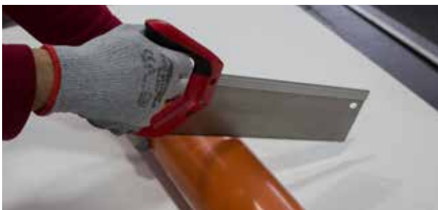
Picture 18: Cutting pipes
