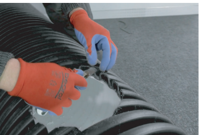
5. Cleaning chips and forming a clear hole
