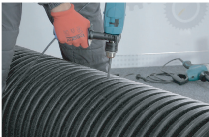
3. Drilling holes for the guided crown saw
