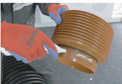
10. Lubricating appropriate connection of sag
