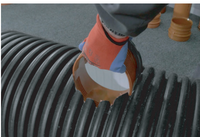
7. Inserting body og sag through pre-prepared opening and setting int in the appropriate position
