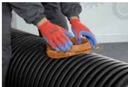
9. Tightening the sag
