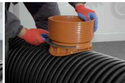
12. Final tightening of sag
