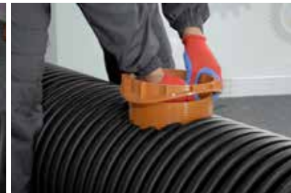
8. setting the spacer ring
