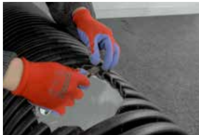
5. Cleaning chips and forming a clear hole
