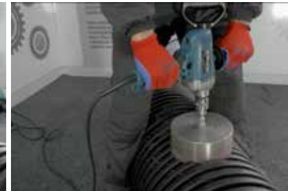
4. Drilling holes with crown saw
