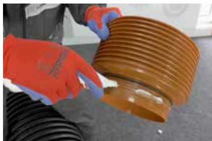
10. Lubricating appropriate connection of sag
