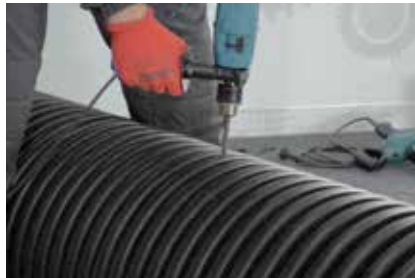
3. Drilling holes for the guided crown saw
