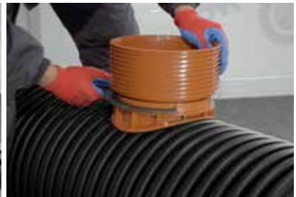
12. Final tightening of sag
