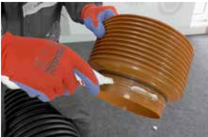
10. Lubricating appropriate connection of sag
