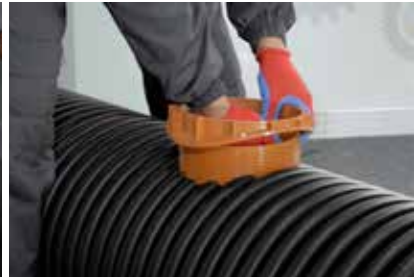
8. setting the spacer ring
