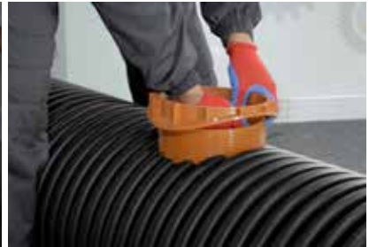
8. setting the spacer ring
