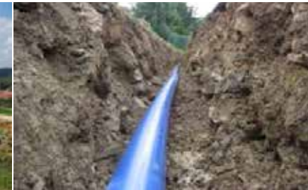
Installation without sand bedding
