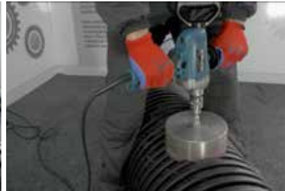
4. Drilling holes with crown saw
