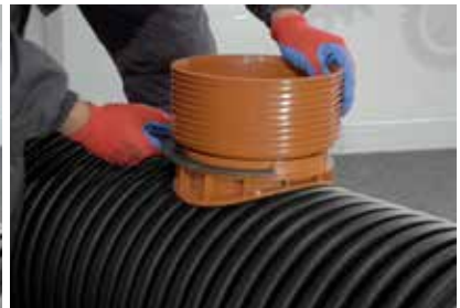
12. Final tightening of sag
