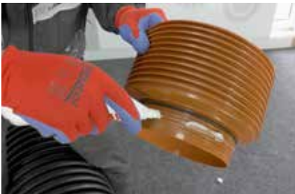
10. Lubricating appropriate connection of sag
