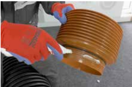
10. Lubricating appropriate connection of sag
