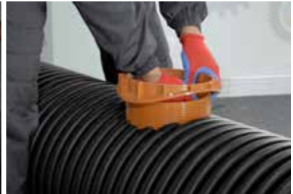
8. setting the spacer ring
