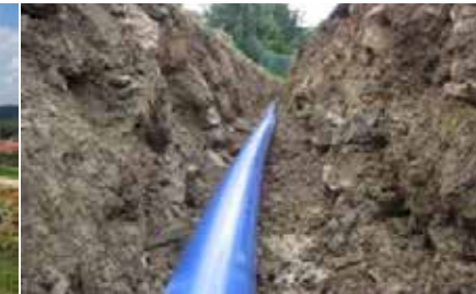
Installation without sand bedding
