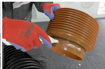
10. Lubricating appropriate connection of sag
