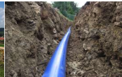
Installation without sand bedding
