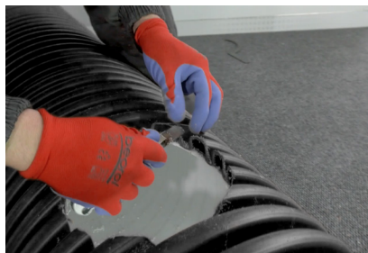
5. Cleaning chips and forming a clear hole
