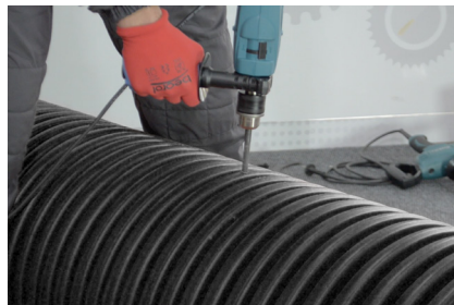
3. Drilling holes for the guided crown saw
